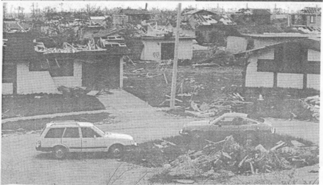
The rebuilding of Homestead, Florida after hurricane Andrew came through is just one roof at a time. Local broker, Randy Pribyl, shares his story of helping do just that looking at the devastation from the top down.
